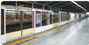
Half Height Type (APG) Half height type screen doors aligned with the location of train doors
