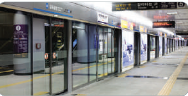
Full-Closed Type Structure of perfectly dividing the platform area and the railway area by screen doors
