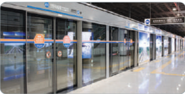
Semi-Closed Type Structure of dividing into the platform area and the railway area by screen doors but there are space between the upper part of the screen doors and the ceiling open
